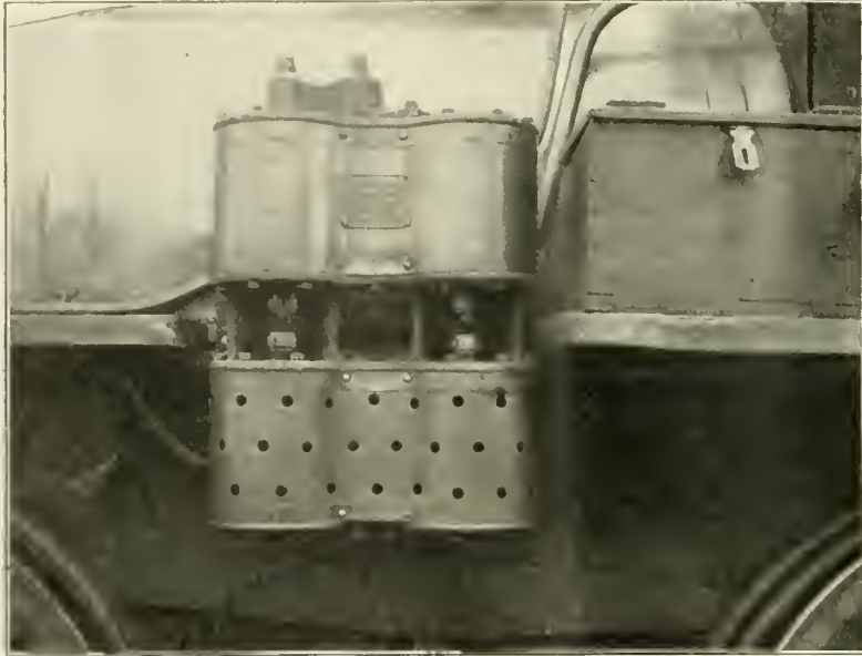
MARSH'S COMPOUND AIR PUMP ON ENGINE.
